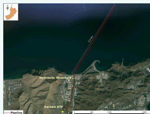
Figure 2: The Azaibah Sewage Pipeline Area [39]
